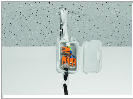
Pendant light connection in suspended ceilings
